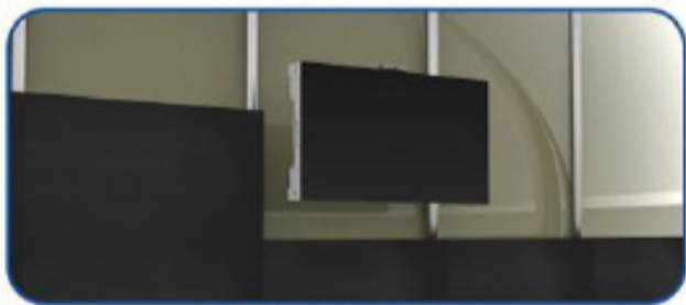
From front installation
