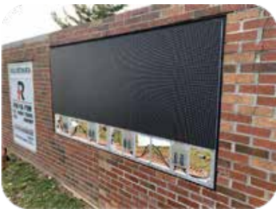
In-wall installation (Utah, USA)
